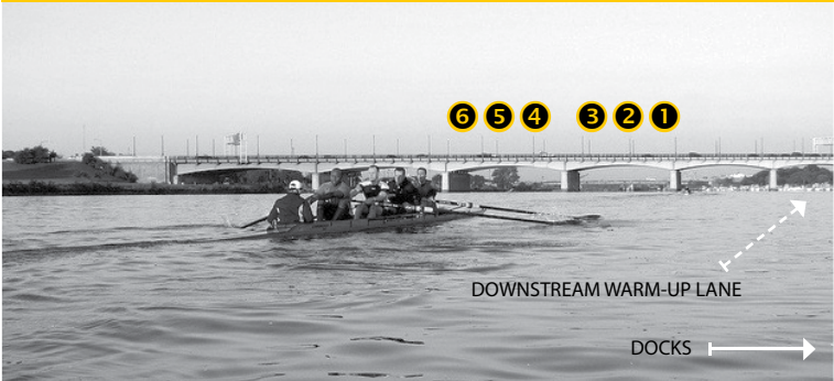
VIEW OF PENN. AVE. BRIDGE AFTER LAUNCHING
