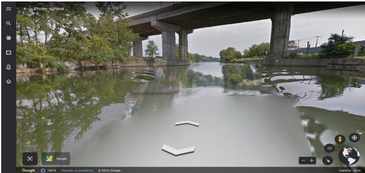
Picture 6c - Obstacle (O2) of the Route 138 overpass - View from the water - Direction Start
